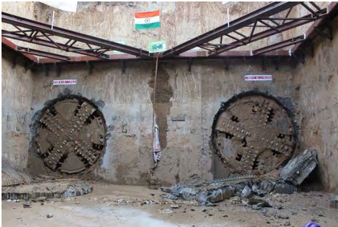
Figure 13: Twin Tunnel Breakthrough marking completion from Apparel Park to Kalupur
