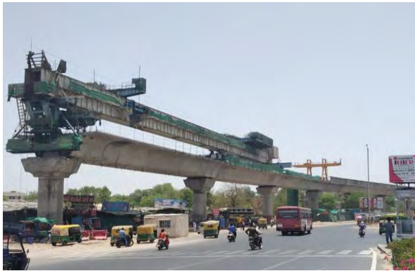
Fig 21: Segment Launching near RTO
