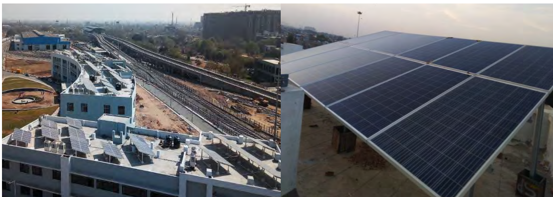
Figure 19 Solar Photovoltaic plant installed on roof of Admin Building in Apparel Park Depot
