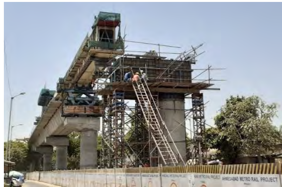
Fig 22 : Segment Launching near Motera
