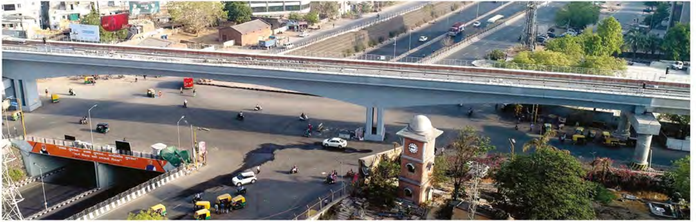
Cantilever Metro Station Bridge at Thaltej
