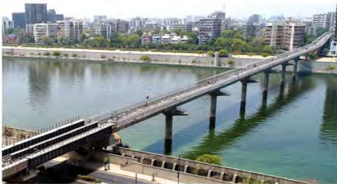
Bridge over Sabarmati River
