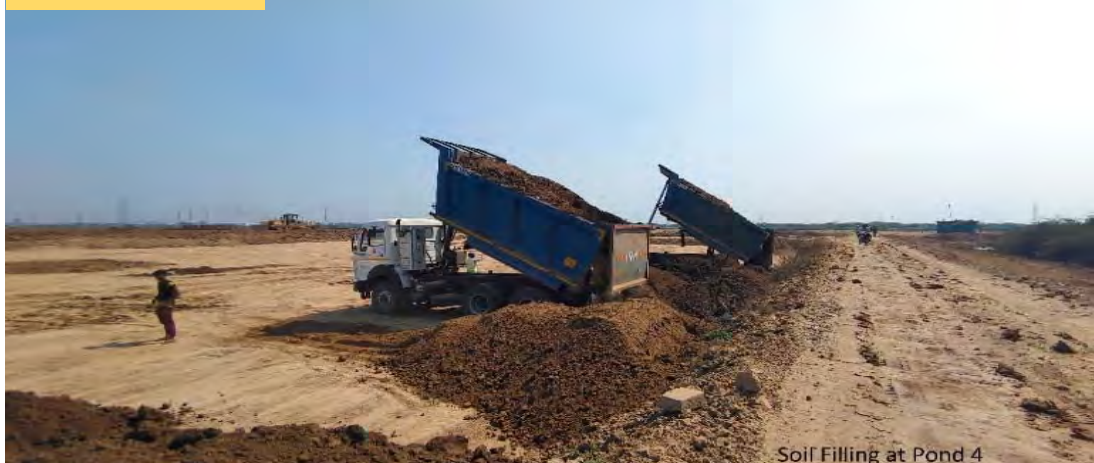
Earthwork in progress
