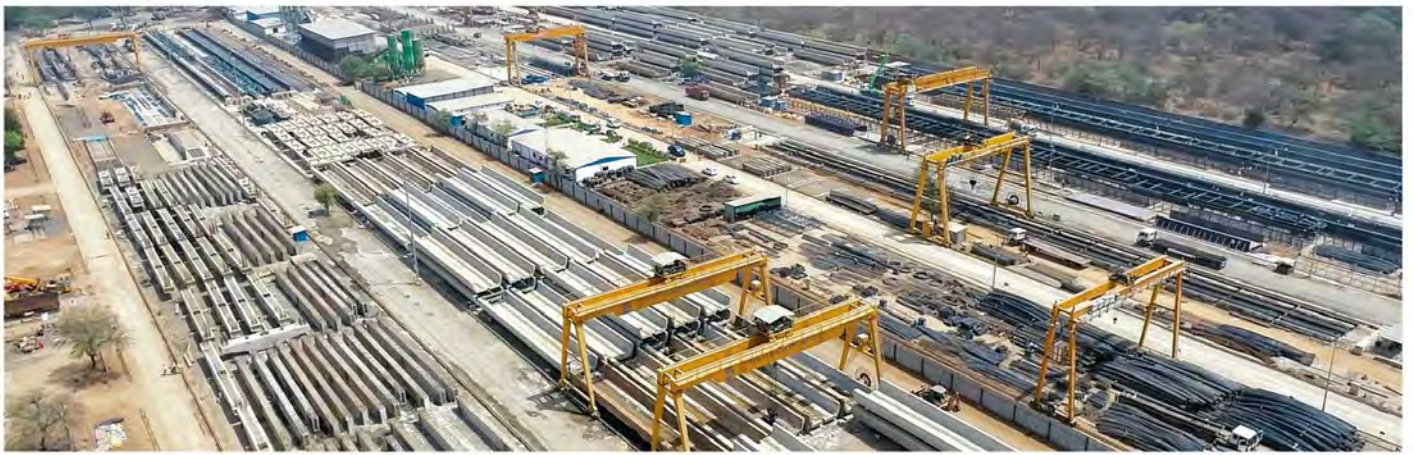
Casting Yard for Ahmedabad Phase-II at Indroda
