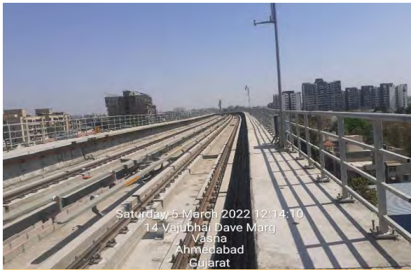
Third Rail Installation (Rajivnagar to Shreyas)
