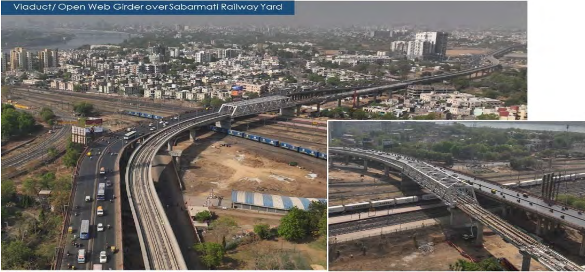
Viaduct/ Open Web Girder over Sabarmati Railway Yard
