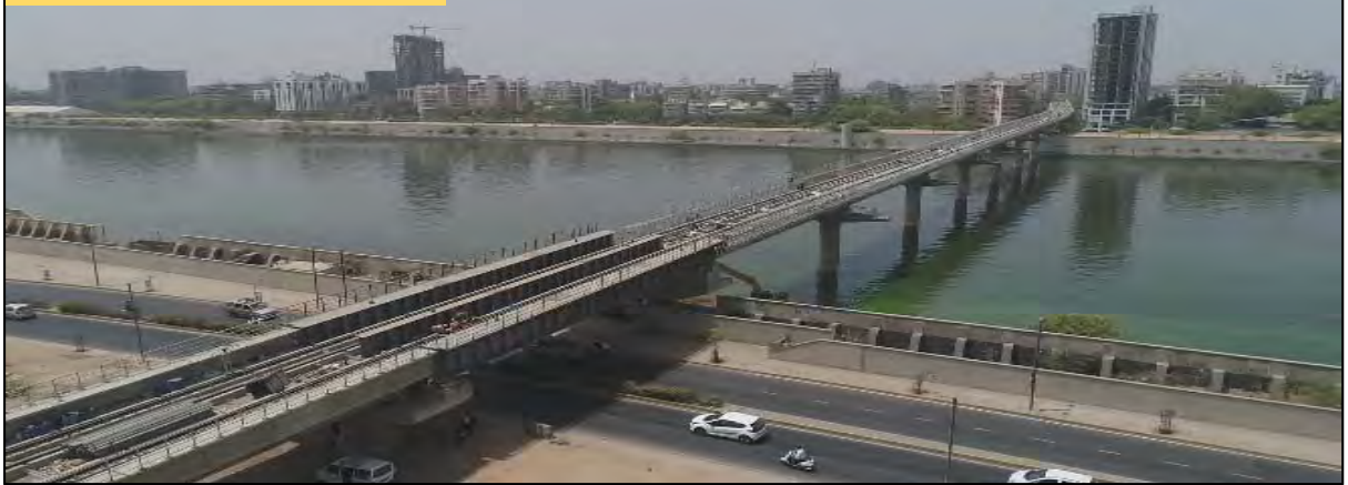
Bridge over Sabarmati River
