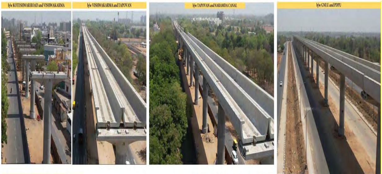
Erection of U-Girder
