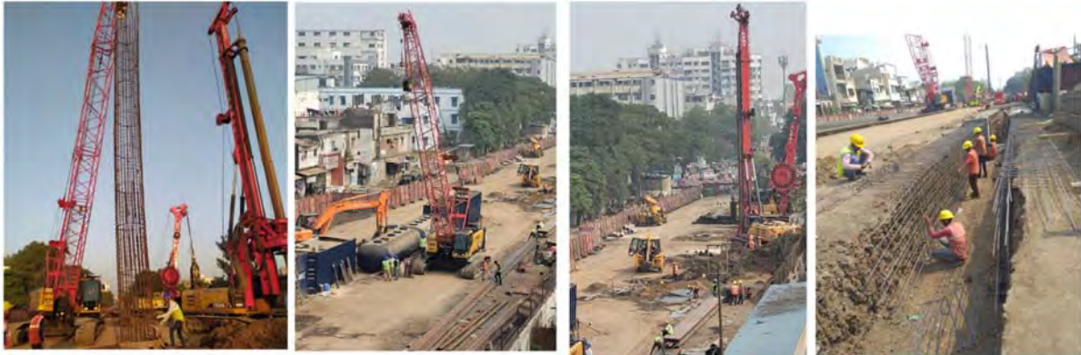
Piling, Guide Wall & Diaphragm Wall Works in Progress
