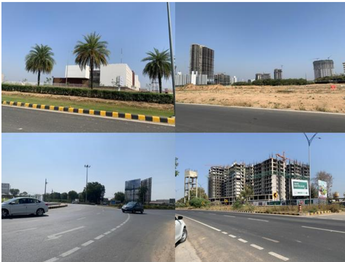
Figure 6.5 : Site Condition: Sabarmati River
