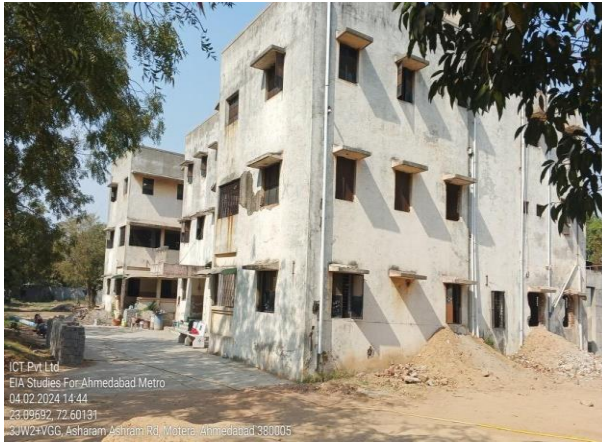
1 Bhera munga School and Hostel
