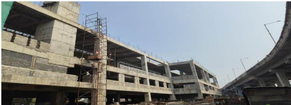
Sabarmati Railway Station - Civil Finishing Work in Progress
