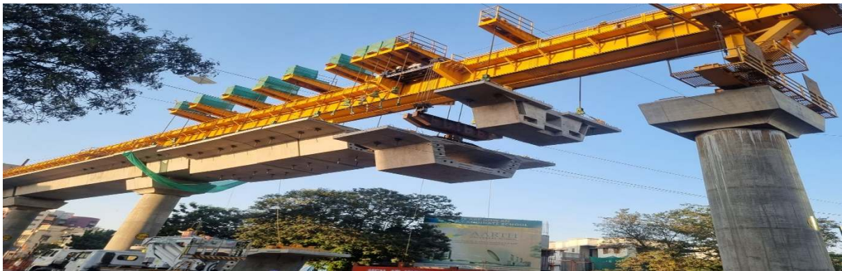
SEGMENT ERECTION
